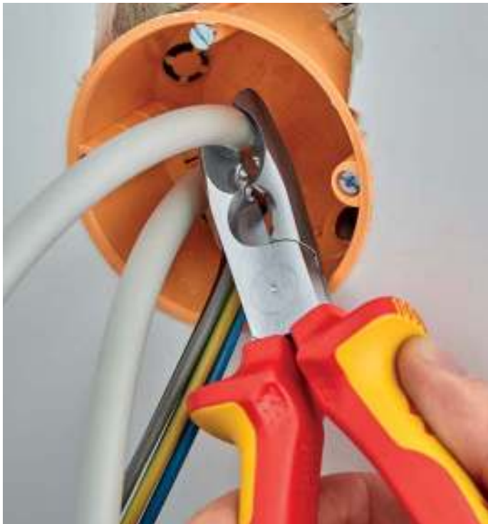
Stripping cable inside deeply mounted junction boxes
